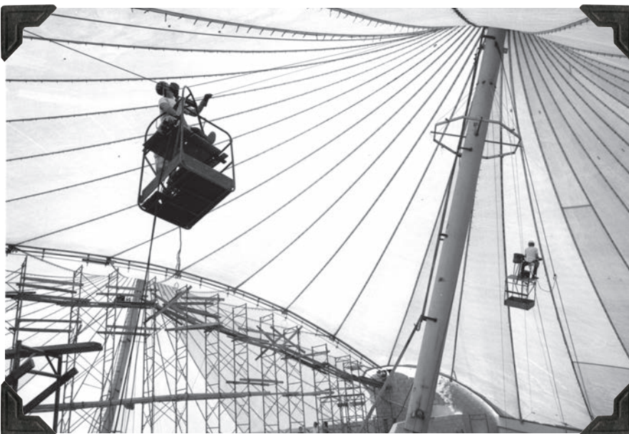
Workers installing support structures underneath the canvas of the Super Tents.
